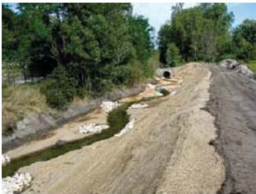
Linear treatment wetland with low flow channel, one week post construction.
