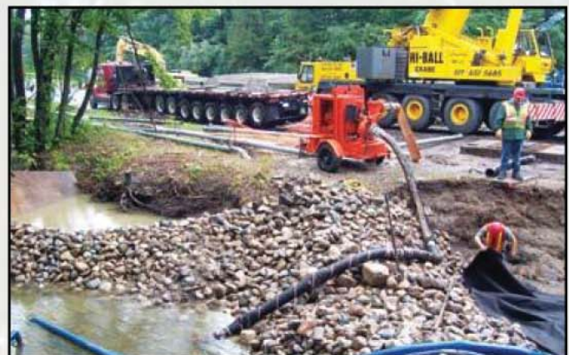
Right: Bank Stabilization along Briarwood Drain
