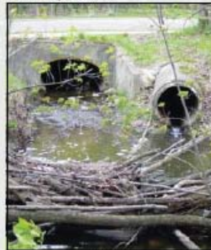
Tree branches and debris form an imperfect and very temporary effort to dissipate effects of high flow.
