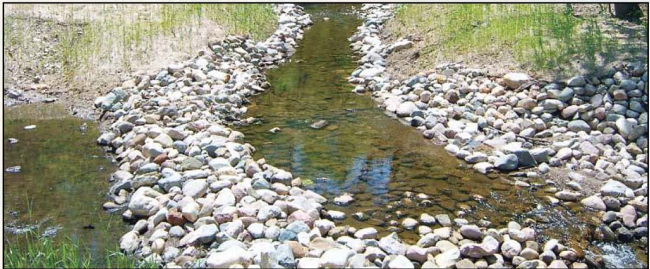
"Steps" along the channel bottom create cascades that improve water aeration.
