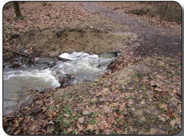
Outlet under the path in Bancroft Park, after leaving the perched wetland located in the middle of the park. Note side-wall erosion. Soon the surface and then the sub-surface of the Esker will be destroyed by this erosion. This flow must stop.
