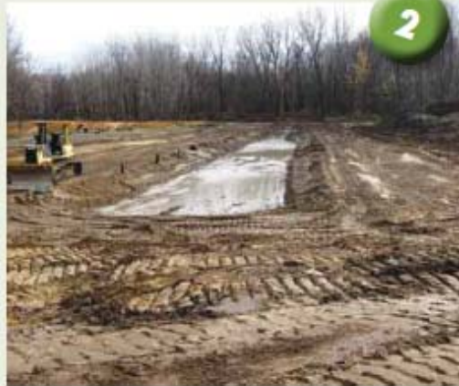
Under-drain system constructed
