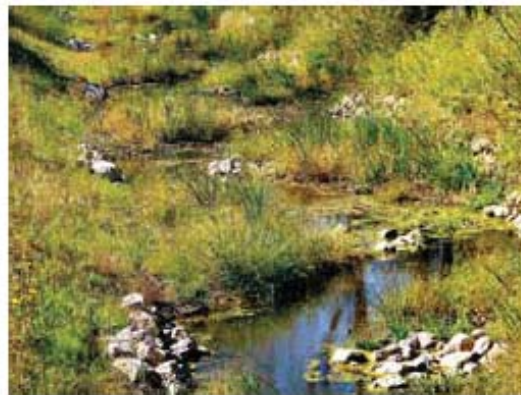
Linear treatment wetland with low flow channel, one year post construction.
