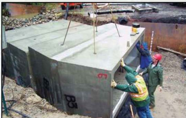
Left: Retrofitting of continuous curvature culvert required precise configuration to harmonize with the pre-existing road profile.
