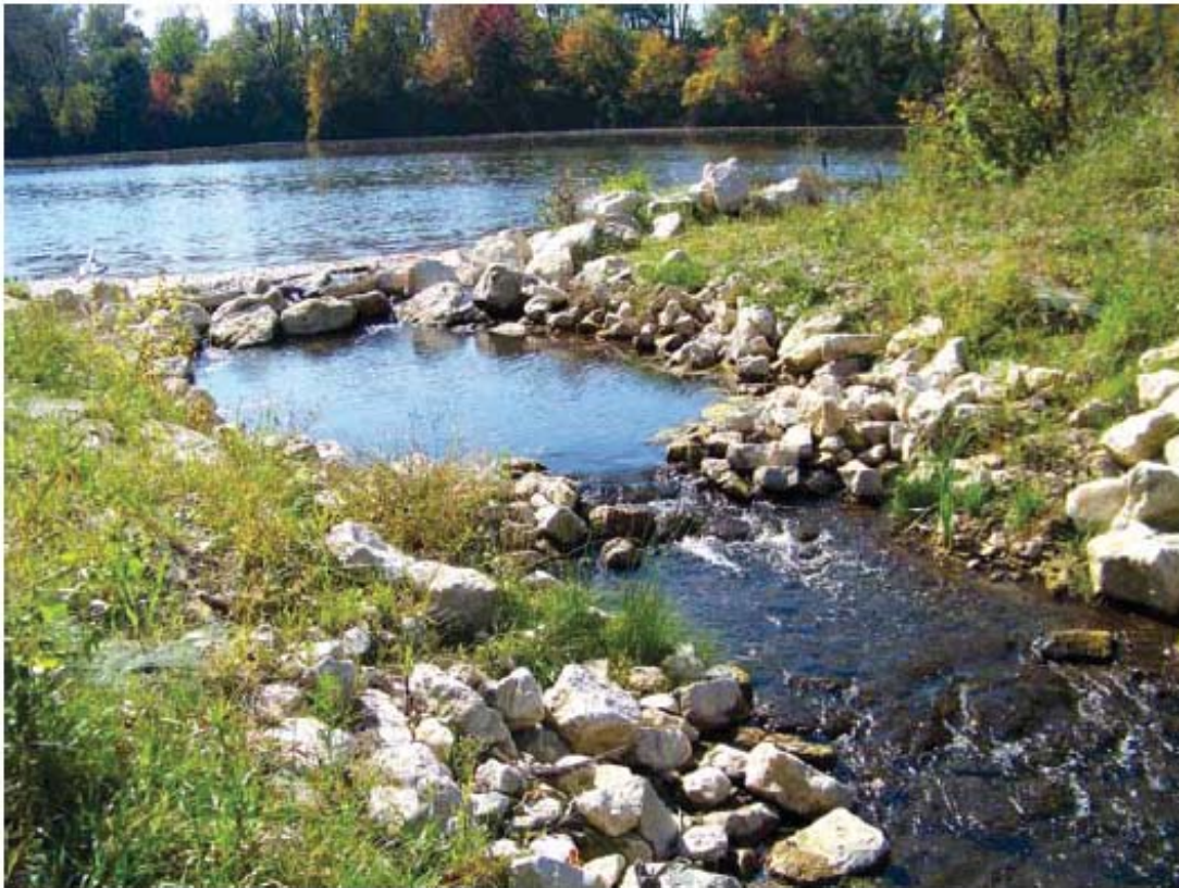
Rock weirs with natural stone riffles at Cedar Lake.
