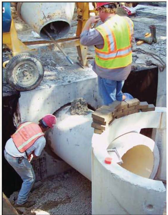
Storm drain fitted into Kinawa Drive culvert.
