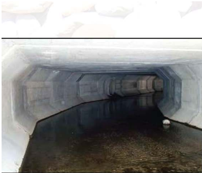
A "natural" stream bottom simulated inside the Kinawa Drive culvert.
