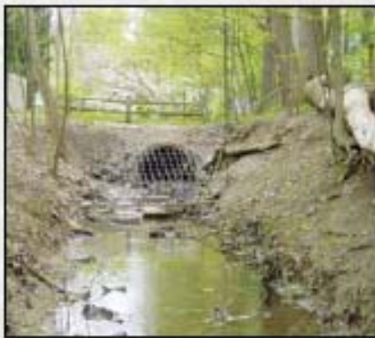
Bank erosion near this 60" storm drain outlet is typical of conditions along the open section of Briarwood drain.
