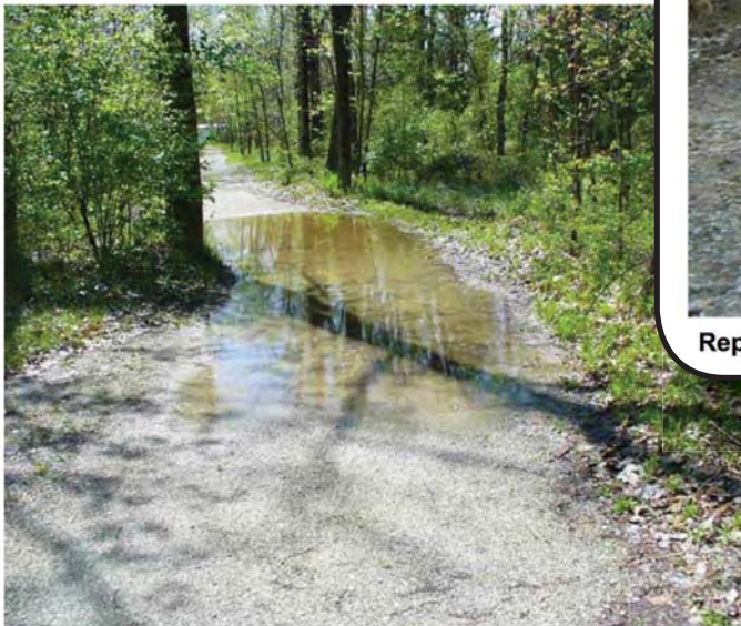
Compacted gravel with fines is not very pervious.
