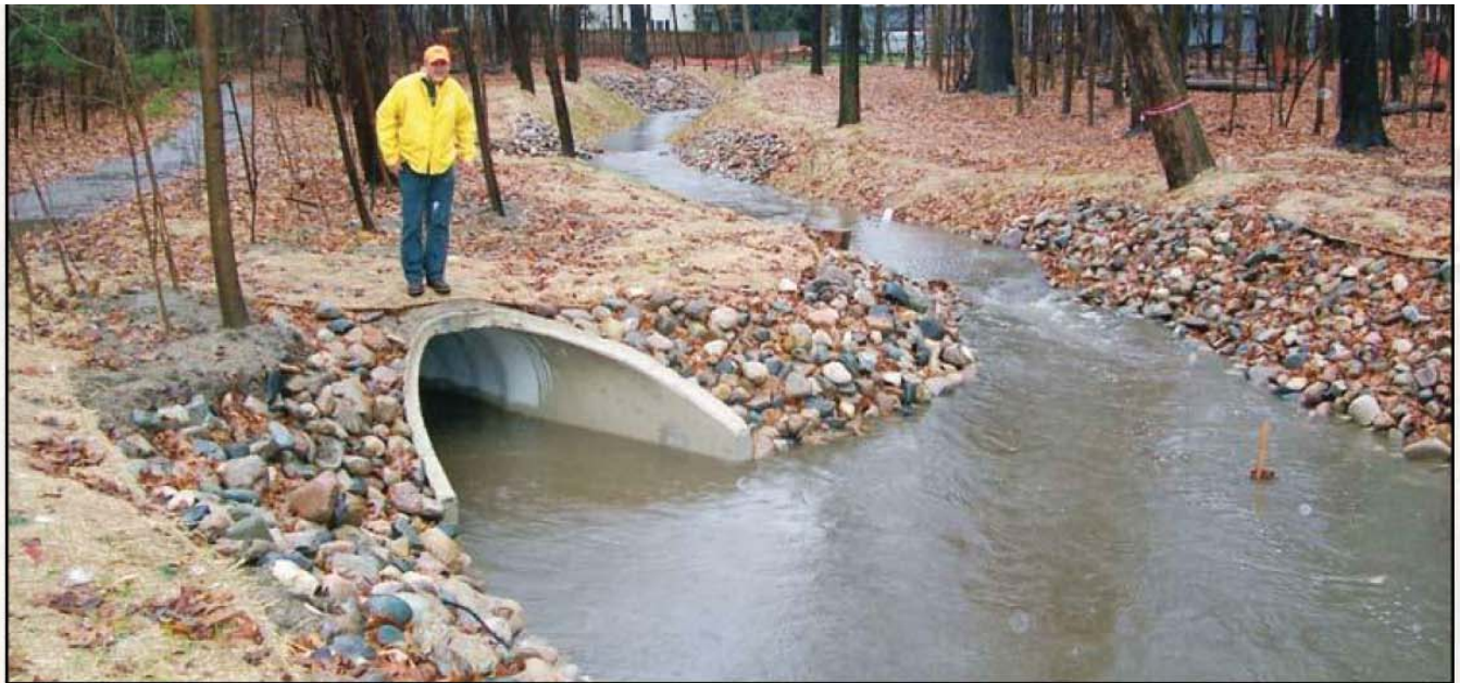
David Solberg of the Ingham County Drain Commissioner's office observes wet weather performance of the riprap reinforcement along Briarwood Drain
