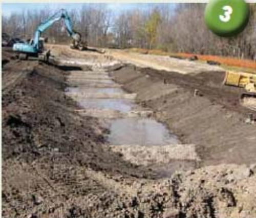
Final shaping and grading
