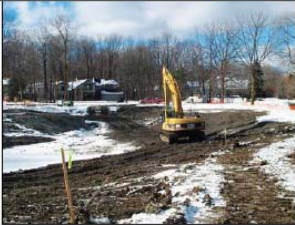
Above: Contractor reshapes the pond to easement boundaries and adds a forebay. Below: The sinuosity visible here will increase stormwater retention time and improve habitat for aquatic life.
