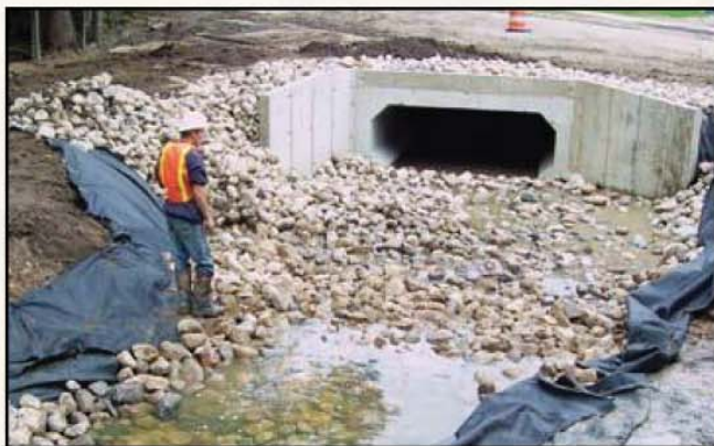
Kinawa Drive culvert outlet configuration vastly improved after construction.
